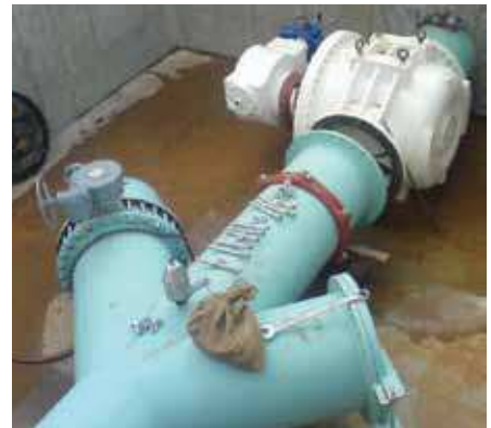
48" (1200mm) Model R-88 couplings used in a water treatment plant, Quary, Utah, USA
