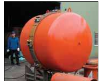
Hydrostatic testing - 72' R-88 coupling
